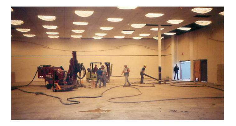
Figure 1. Judy Company providing compaction grouting services inside a building.
