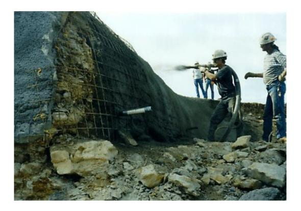
After the mesh is in place, holes are pre-drilled and friction stabilizers are driven in place. The anchors are split tubes that are squeezed as they are installed like alarge automotive roll pin. Ingersoll Rand or Friction-Lok, Inc. manufactures the anchors. Typical spacing is a 5 to 7 foot square pattern depending on rock conditions. Various sizes and lengths are available, the most common requiring a 1.75 diameter hold with a length of 4 to 6 feet.
