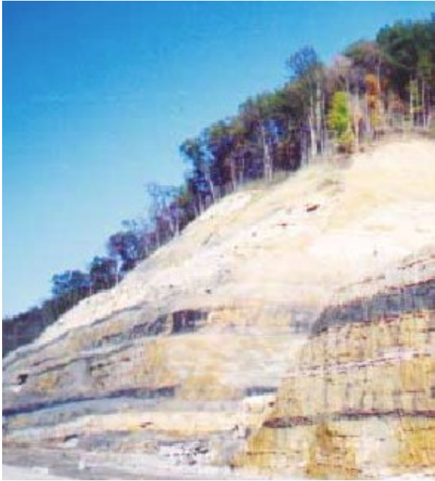
A retaining wall in Kentucky was stained after curing to create a more natural look.
