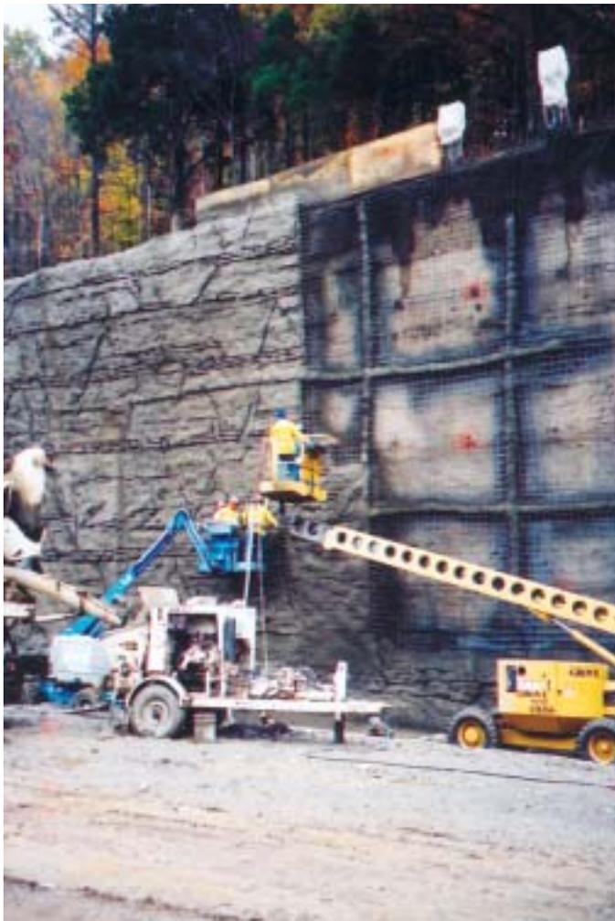
The Judy Company uses a Schwing trailer-mounted concrete pump with line system to apply shotcrete. Decorative landscape rock artisans are brought in to achieve a more realistic aged rock look on a shotcrete surface in Kentucky. This process must take place immediately after the shotcrete is sprayed onto the excavated wall.
