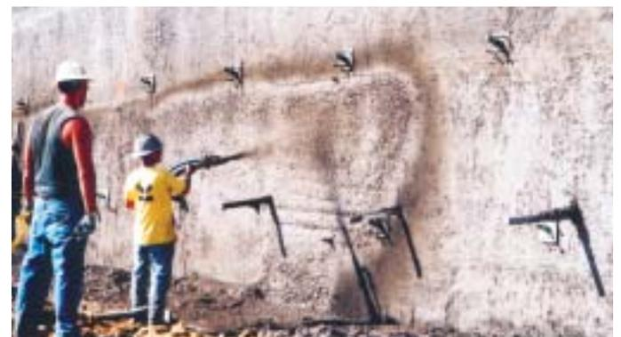
Reinforcing steel is applied and the face is shotcreted. Behind cast-in-place concrete finish, shotcrete can be left rough or lightly troweled.
