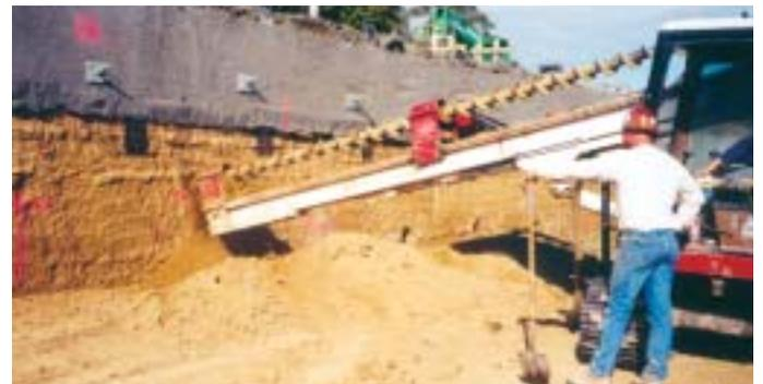
Holes are drilled into the excavated face typically measuring 6 to 8 inches in diameter in soil, and 3 to 4 inches in rock.
