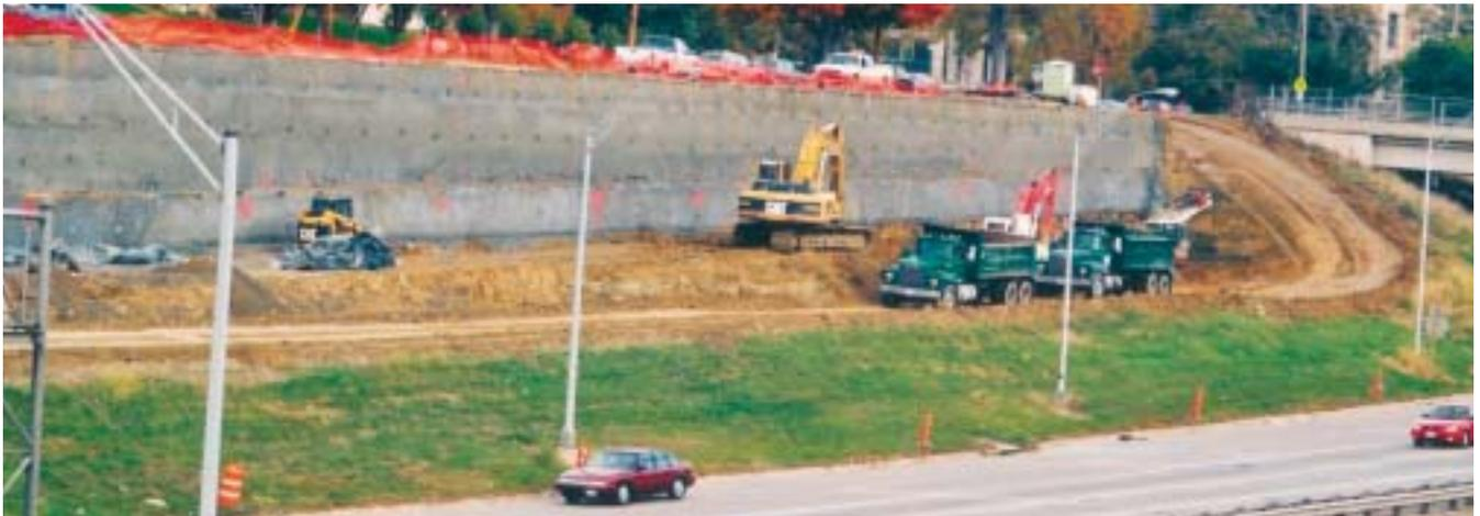
About 63,000 feet of retaining wall was constructed off I-235 in Des Moines using the soil-nailing method. Upon completion, the walls were covered with pre-cast panels.
