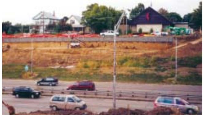
The first bench of the Des Moines retaining wall project is completed. Soil contractors only cut as long a bench as crews can complete in a 24-hour period, to prevent collapse.
