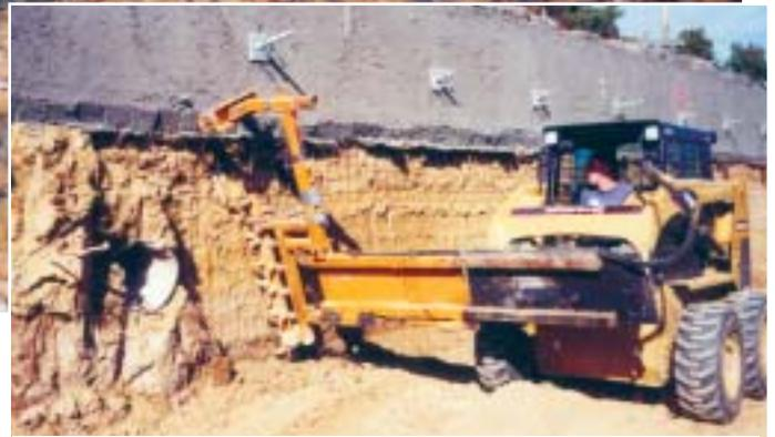
A cutter attachment on a skid steer is used to create the second bench.
