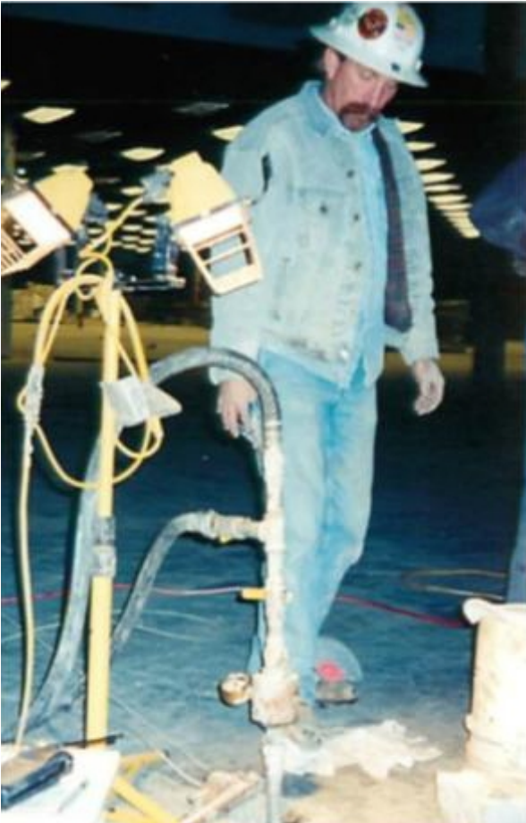
Moving up grout injection pipe Employee monitoring grout injection pipe
