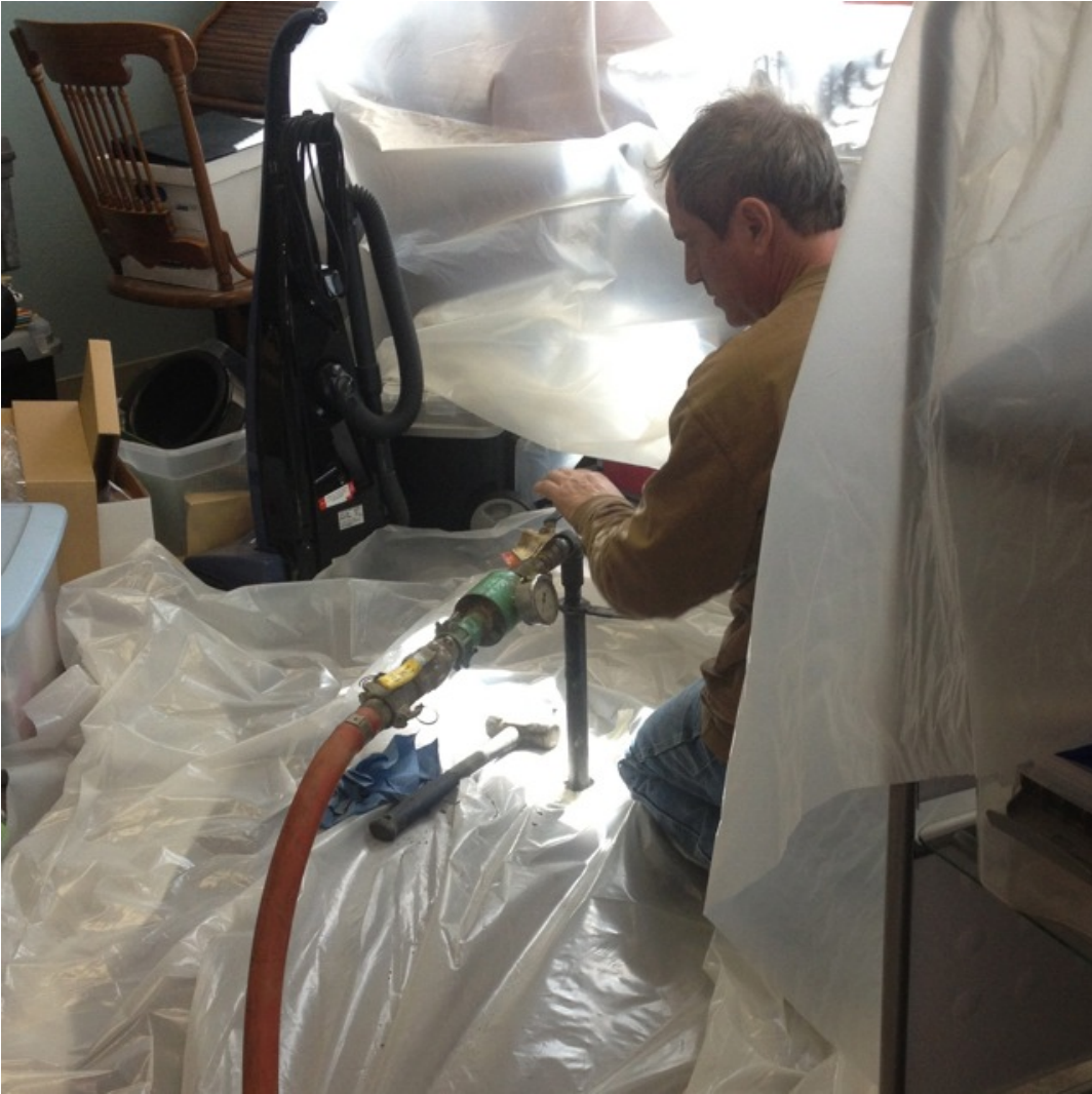
Figure 1. Pressure Grouting Inside a Building
